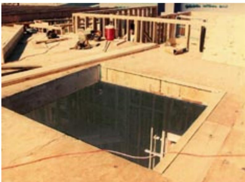
Use guardrails or covers to prevent workers from falling through floor holes.
