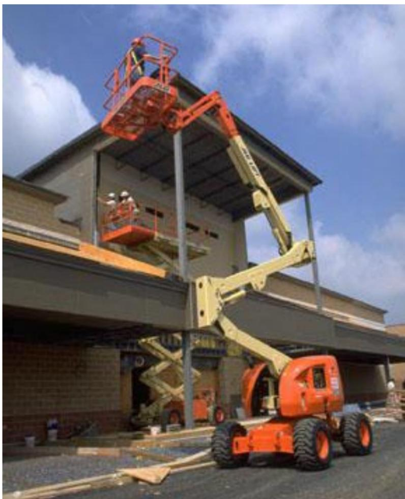
**Warning!** Aerial lifts are designed to operate on level, solid surfaces where they will not sink or slide.
