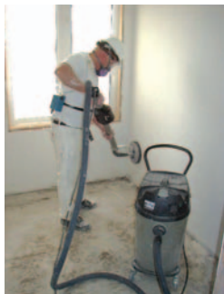
Figure 2. Shrouded ventilated rotary sander attached to vacuum.
