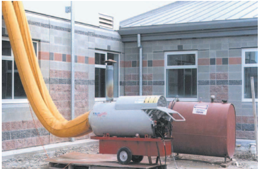
This oil-fueled indirect-fired heater vents emissions outdoors while heated air (free of emissions) is ducted indoors.
