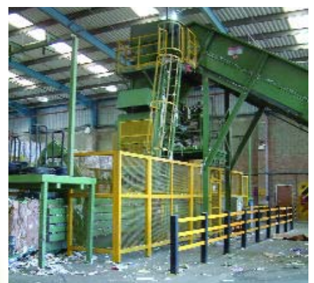
Guarded needlepit, bale ejection mechanism, access ladder to top of conveyor, and platform. Note barrier protection to prevent vehicles striking baler and conveyor
