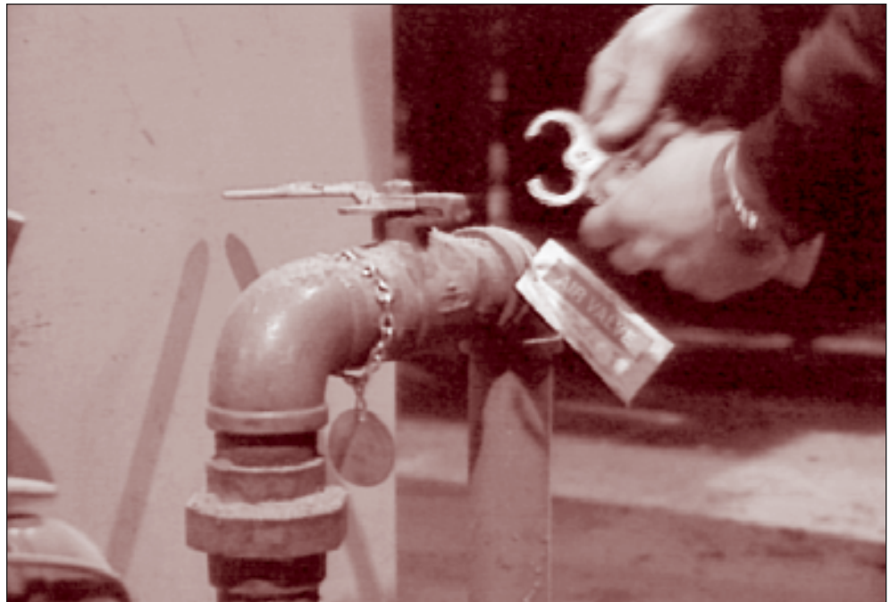
Apply a personal lock after the valve has been closed.
