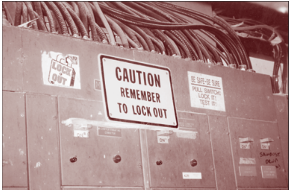
Post lockout notices as part of your lockout system.
