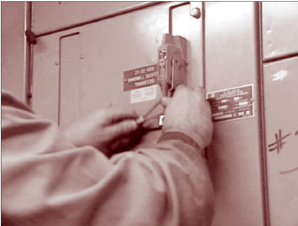
Use a cable to lock out several disconnect switches.
