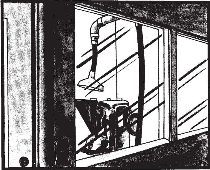
“Dusty” work area isolated from “clean” area
