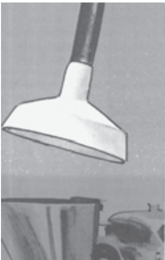
Dust collection duct near source
